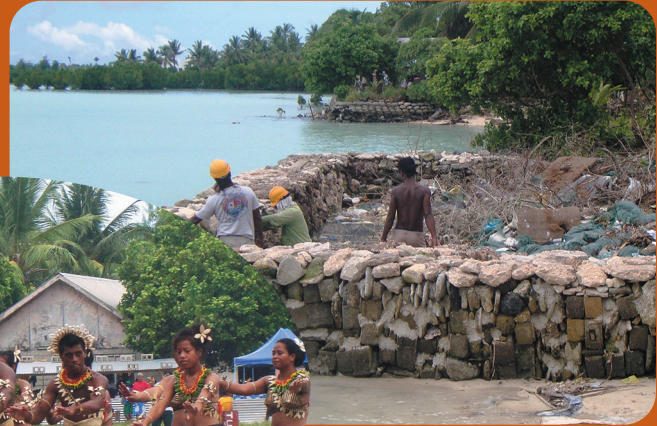
Constructing a sea wall, Kiribati
